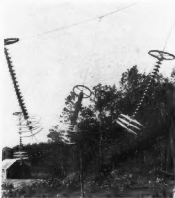
The klydonograph furnished much valuable information on the characteristics of natural lightning and switching transients in the early field investigations.
